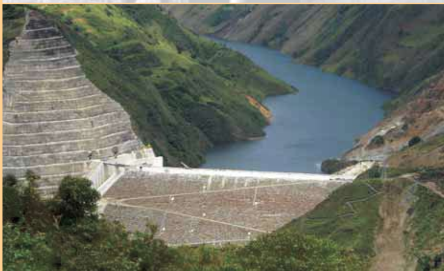
Mazar Hydroelectric- Project - EkBagor
